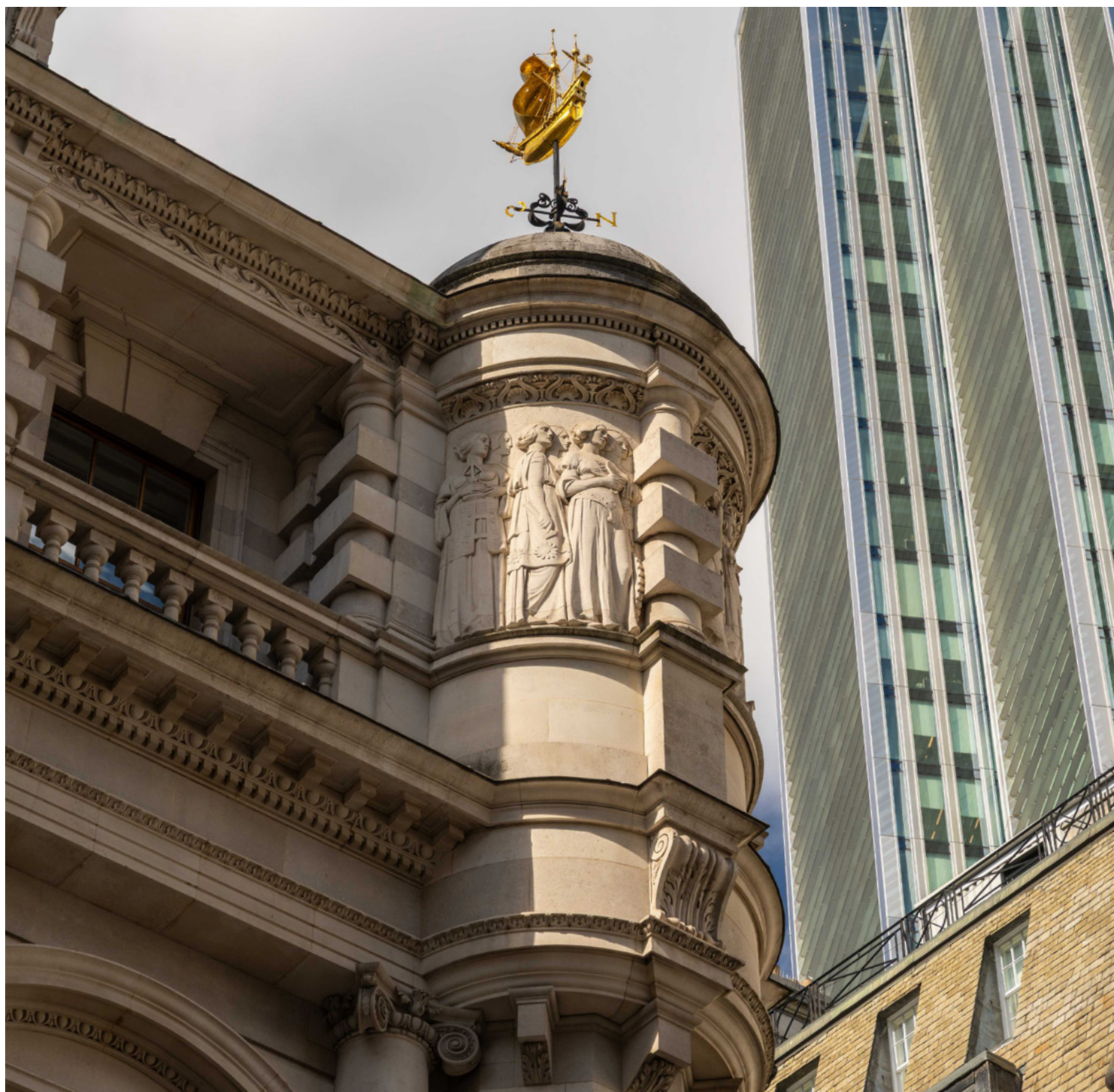
Left: A tourelle at the corner of Lloyd's Avenue is a brass carrack-shaped weathervane by Hardman & Co.
